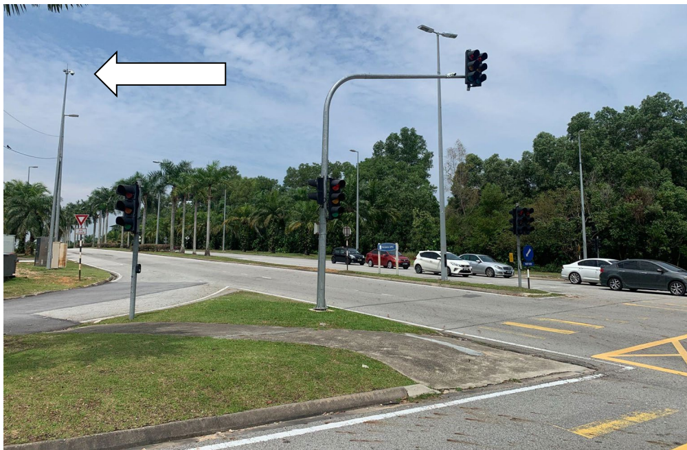
Figure 5. CCTV position at J9 (Jalan Impact)
