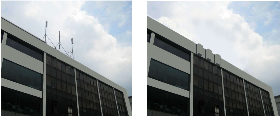
Figure 3. Design using concealment panels
