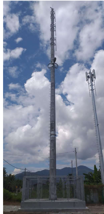
Figure 6. Concrete monopole
