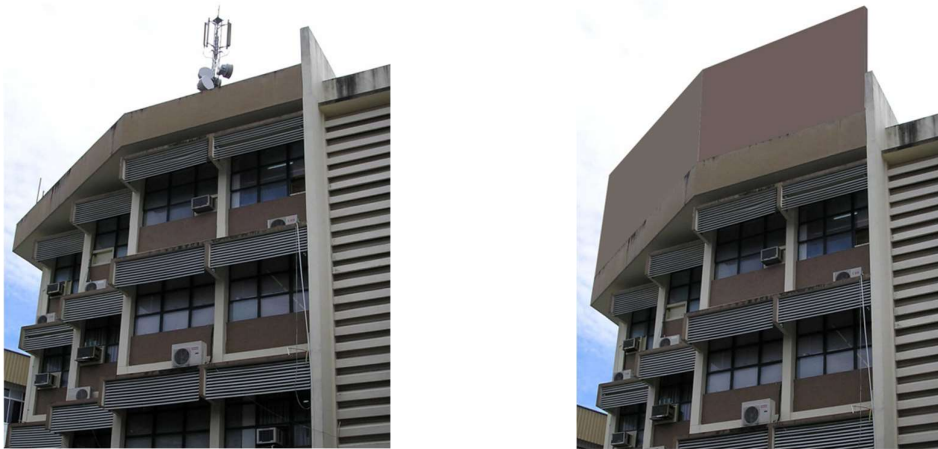
Figure 4. Roof top concealments
