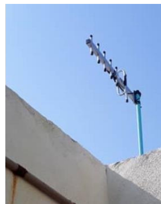
Figure 1c. Receiver node located on the rooftop of Central Lectures Complex in UMT
