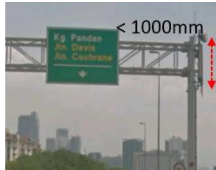
Type B1 - panel antenna mounted at retrofit or existing structure
