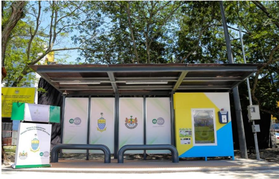
Figure 7. Example of Type D2 installation
