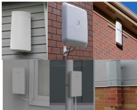
Type B2 - panel antenna mounted at the building wall facade
