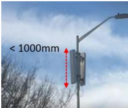
Type B1 - panel antenna mounted at retrofit or existing structure
