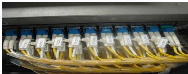
Figure 64. Sample of recommended tagging system
