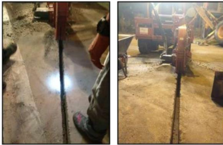
Figure 8. Example of road cutting machine
