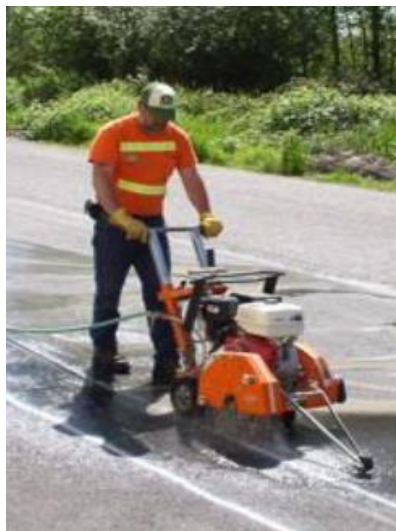
Figure 2. Cutting of asphalt by using road cutting machine
