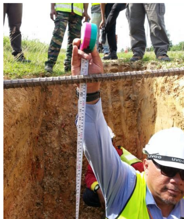
Figure 3. Sample depth of trench measurement
