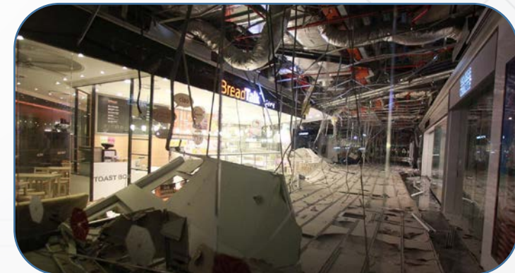
Fig: Ceiling collapse due to cable rest on false ceiling
