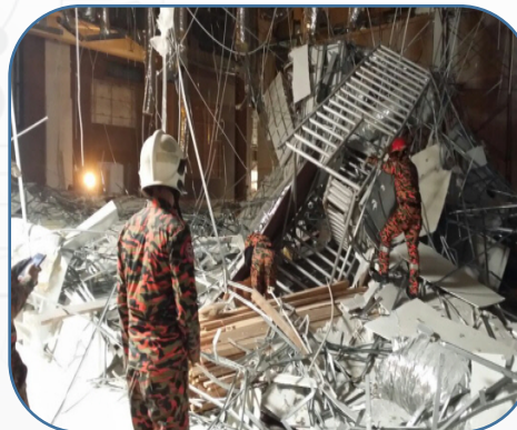
Fig: Ceiling collapse due to cable rest on false ceiling
