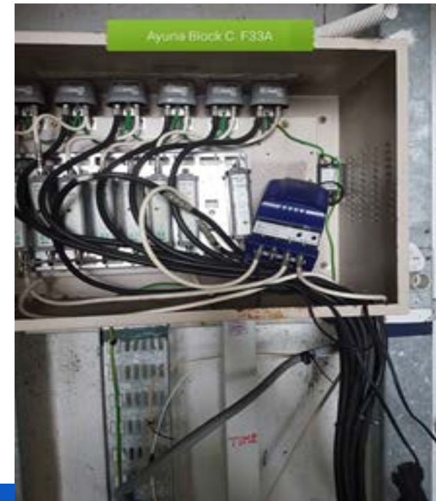
Figure 4. Recommended Head-end equipment arrangement (wall mounted type)
