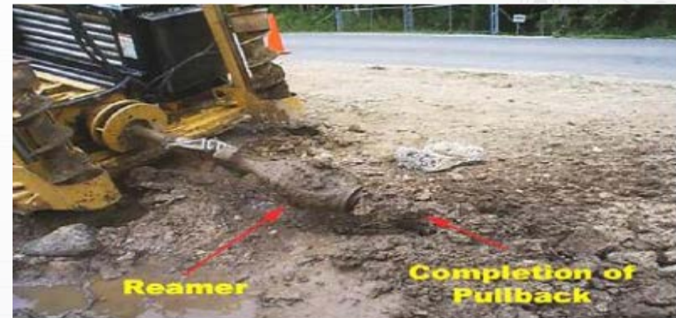
Figure 12. Reamer during completion of pullback process
