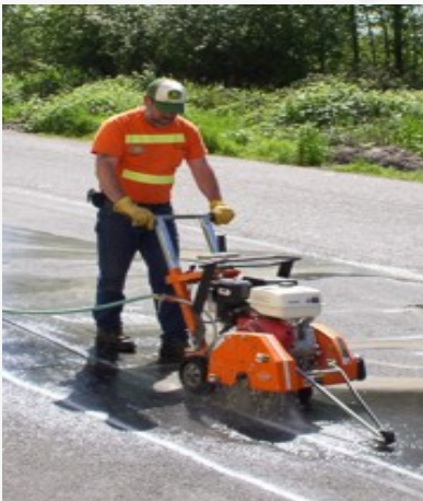
Cutting of asphalt layer using road cutter
