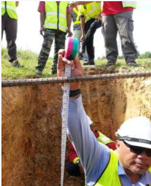
Measurement the depth of trench excavation
