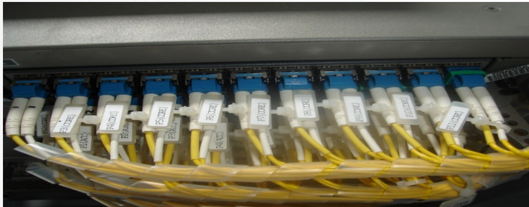
Sample of recommended Tagging System
